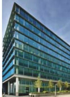
2 Kingdom Street, W2: 26,000 sq ft let to Staitoil
